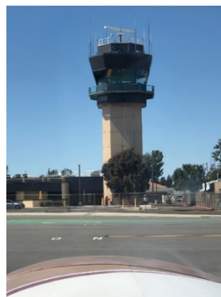
Control tower completely empty!
